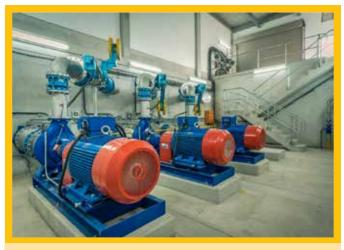
FIGURE 11: Leliefontein Pump-As-Turbines installed, with space for future unit in background
