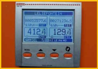
FIGURE 8: Bi-directional power meter at Leliefontein PAT
