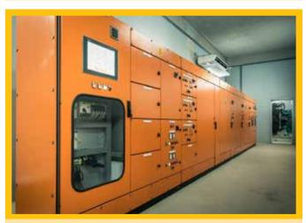
FIGURE 10: Leliefontein PAT Motor Control Centre
