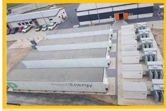
FIGURE 3: 10 MW Battery Installation, Texas US19
