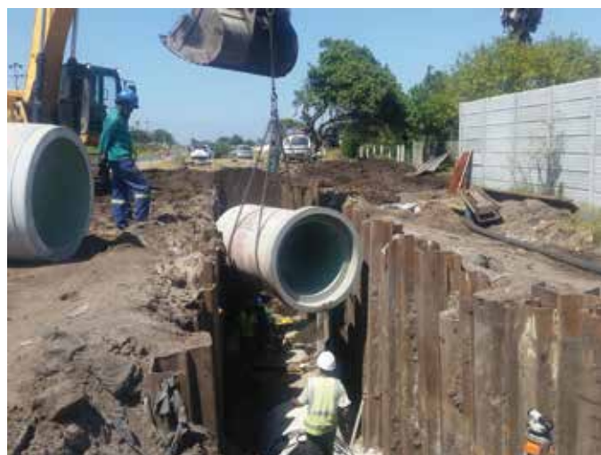
FIGURE 5: Construction of gravity sewer pipeline using the interlocking steel sheet piles
