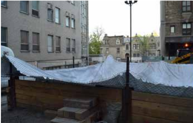
FIGURE 6. Shaft cover used to limit fly rocks and blast mats used to reduce air-overpressure
