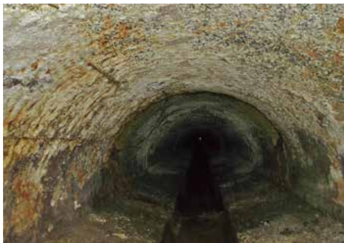
FIGURE 7: Severe corrosion just downstream N2
