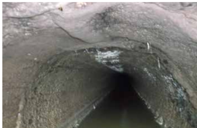
FIGURE 8: Swelling due to corrosion of FC pipe
