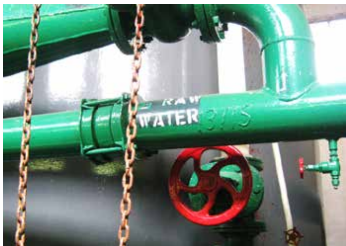
FIGURE 6: Labelling of pipework at Kwa-Mashu WWTW
