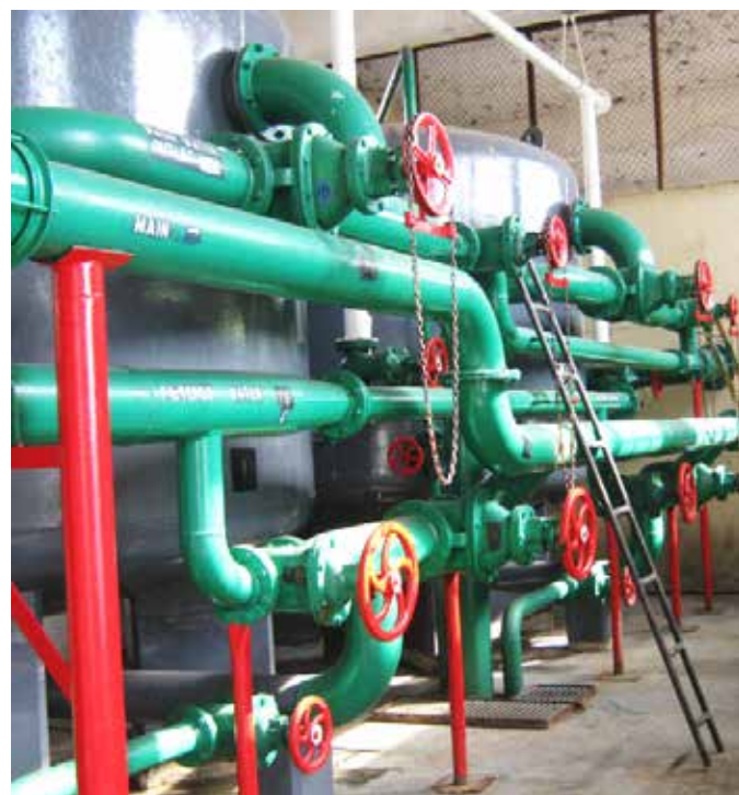
FIGURE 1: Bank of pressurised sand filters located at Kwa-Mashu WWTW, eThekweni Municipality
