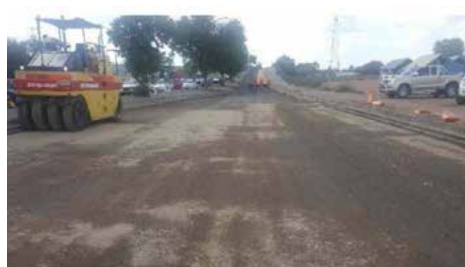
FIGURE 19. Compaction of the BSM
