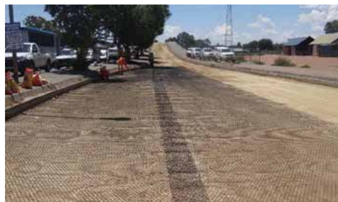
FIGURE 17. Installation of the Triaxial Geogrid
