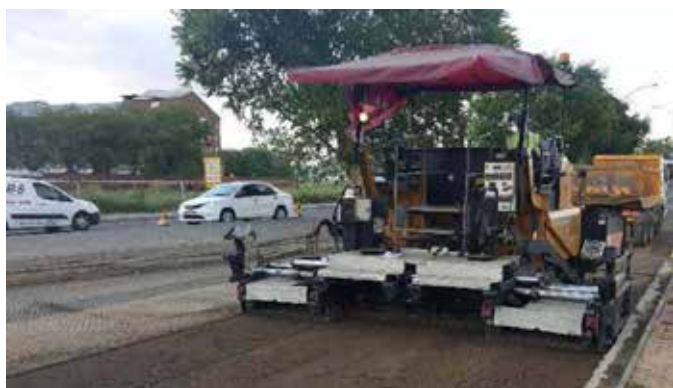
FIGURE 18. Paving of the BSM
