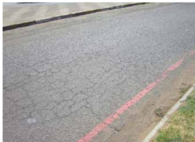
FIGURE 11. Distressed Pavement
