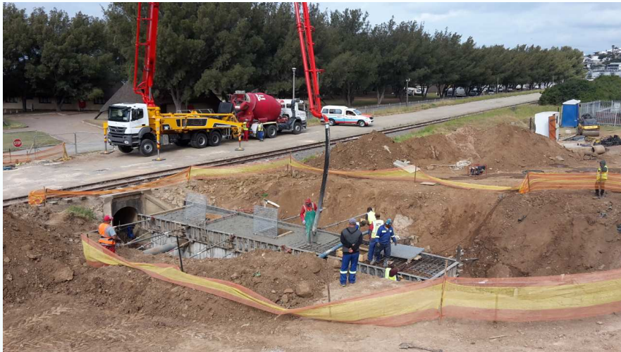
Construction of Railway Stilling Basin
