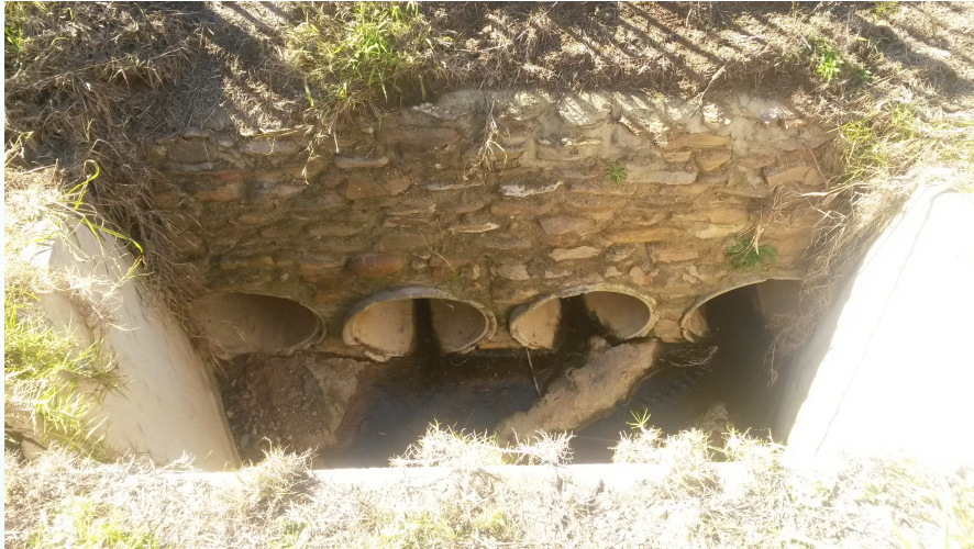
Before Photo of Transition to 4 x 750mm Pipes at Railway Culvert Outlet.
