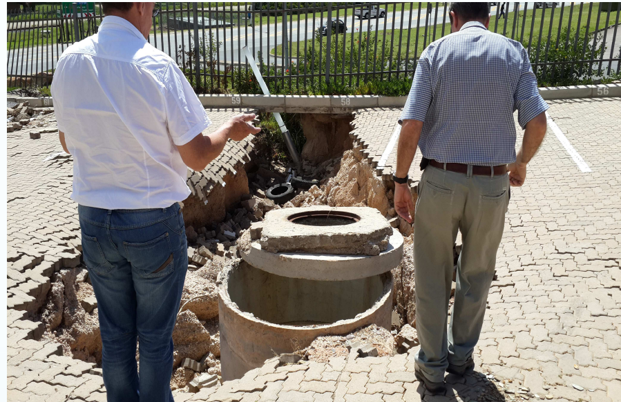
Damage to the parking area at the development
