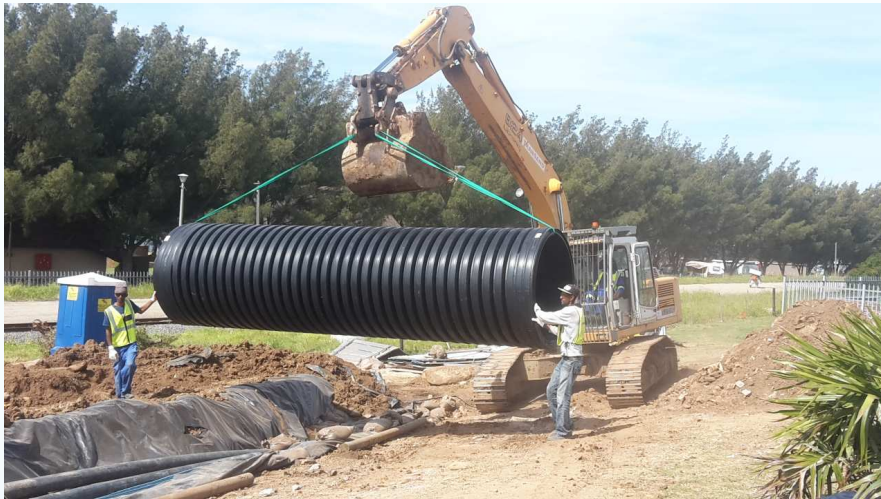
1400mm ND Pipe laying in progress
