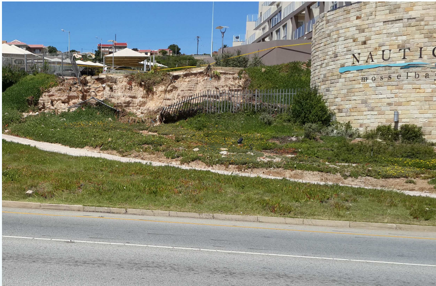
Damage to the raised parking area
