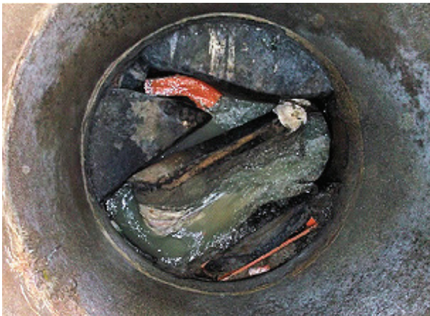
FIGURE 5 Broken benching & supercritical flow
