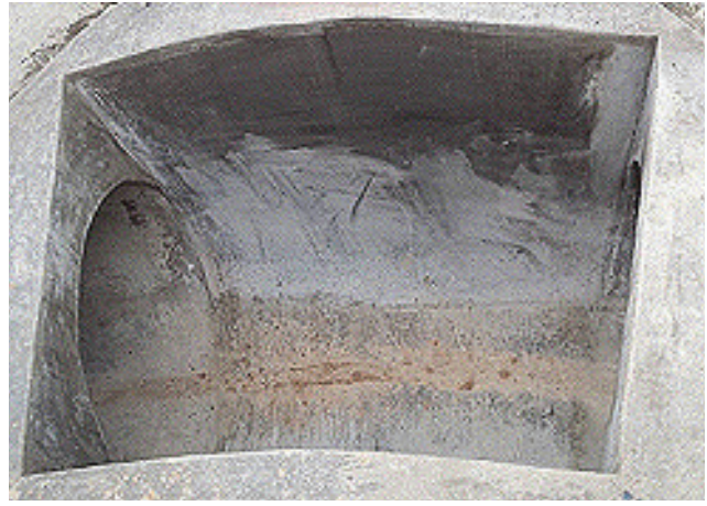
FIGURE 4 Correctly formed benching
