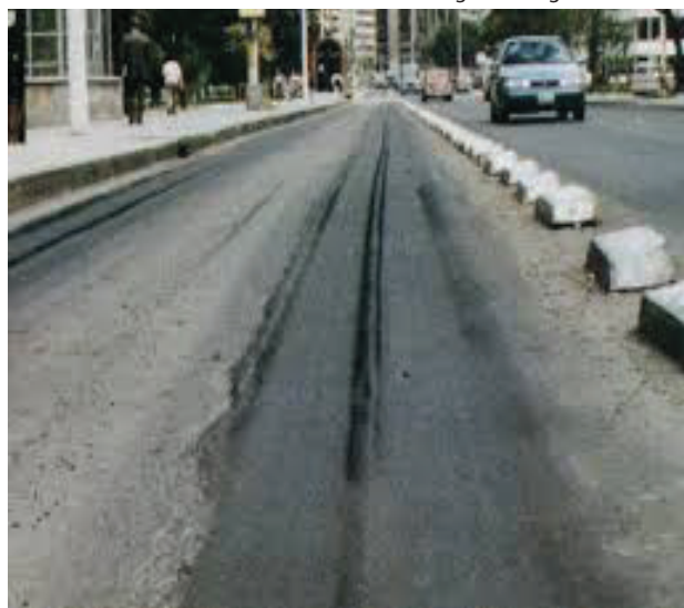
FIGURE 1 Channelized bus lane traffic resulting in rutting
