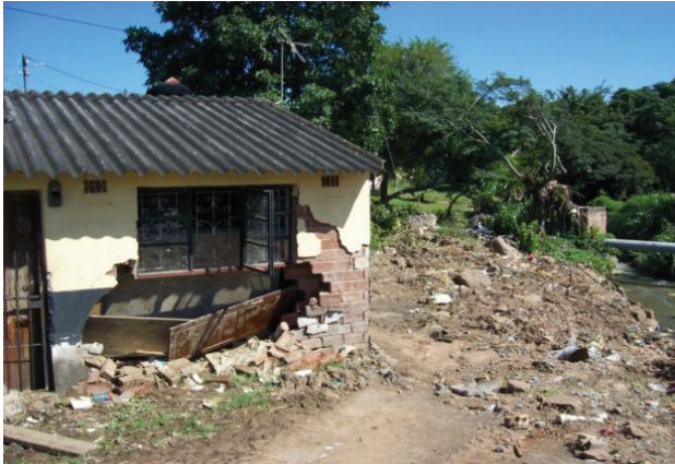
FIGURE 4 This house is situated upstream of a crossing that blocked and the upstream depth of water caused the house wall to fall inwards
