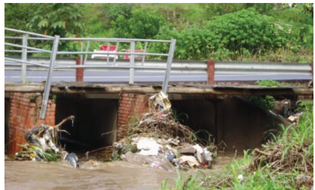
FIGURE 16 Mugabe Road culvert with debris build up
