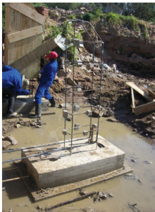
FIGURE 25 Base cast for the debris walls
