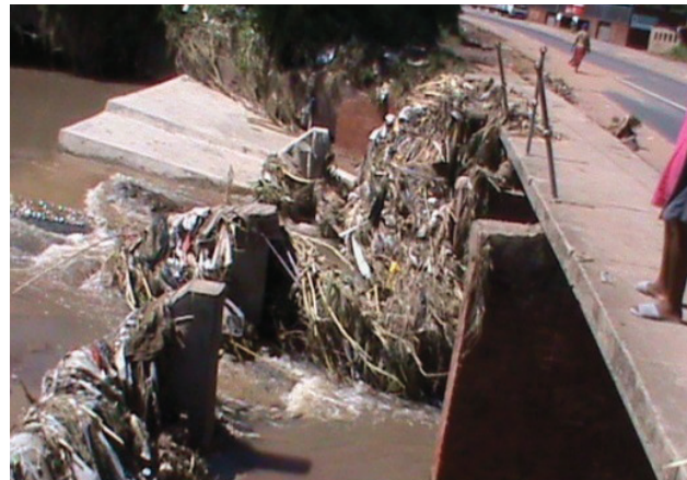
FIGURE 37 Debris build up while the one debris wall was missing
