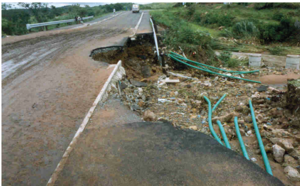
FIGURE 6 The overtopping of the culvert crossing due to a blockage caused damage to the road and services
