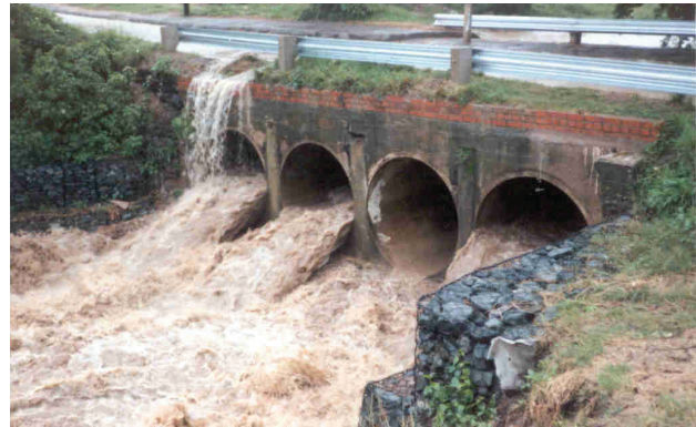
FIGURE 2 The downstream view of the multicellular pipe culvert in Fig.1 during a flood flow showing the reduced flow capacity due to the blockage of the culvert
