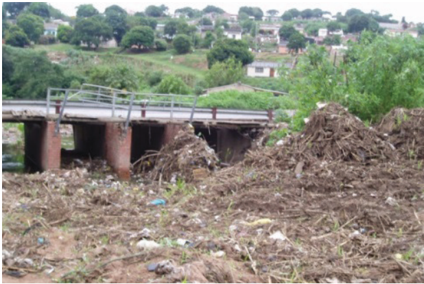
FIGURE 18 Mugabe Road culvert with debris build up
