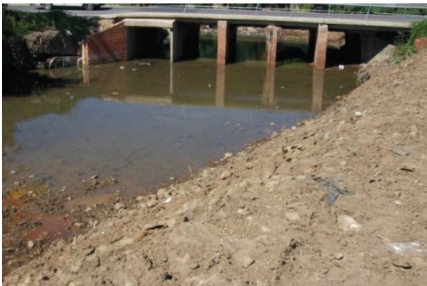
FIGURE 20 The upstream silt has been removed and the additional cell added
