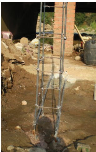
FIGURE 22 Reinforcement for the debris wall dowelled into the inlet slab
