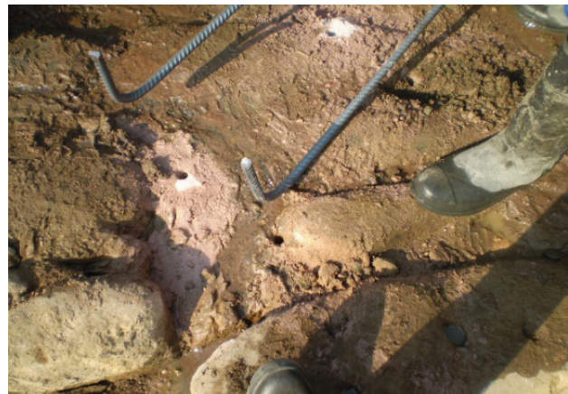
FIGURE 21 Dowel holes for reinforcement into the bedrock
