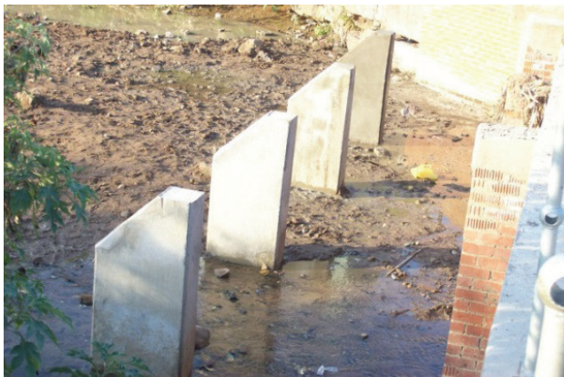
FIGURE 28 Completed debris walls
