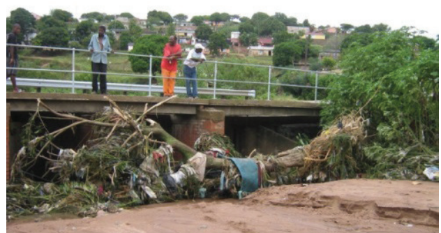
FIGURE 17 Mugabe Road culvert with debris build up – Note the build-up of silt upstream of the culvert
