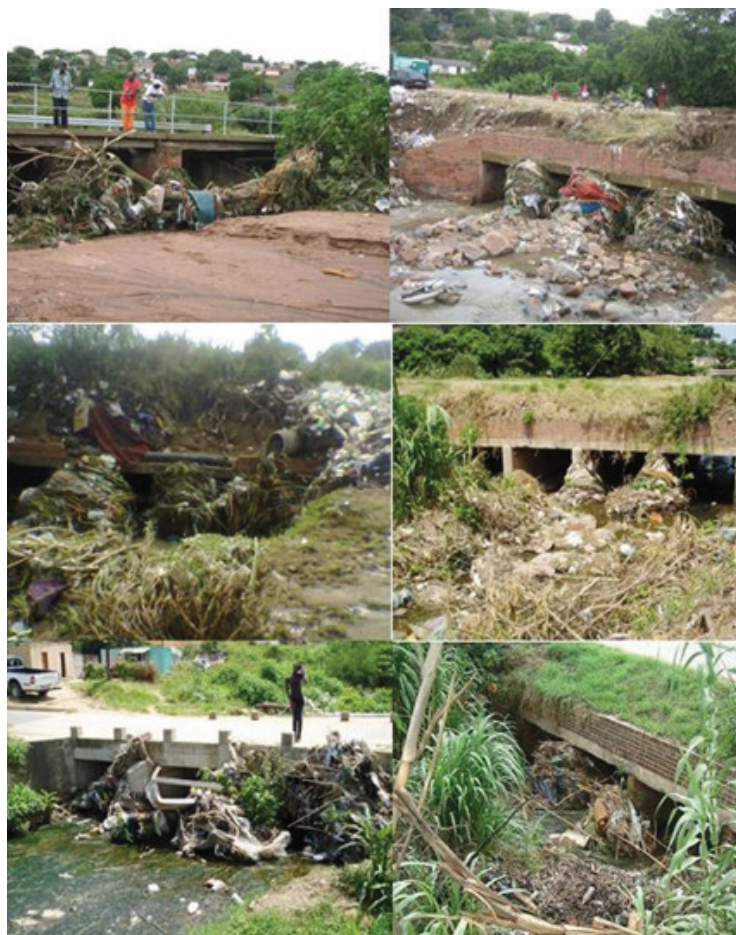
FIGURE 3 Typical blockages of multicellular box culvert crossings - notice the large amount of alien vegetation forming the blockages
