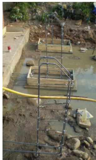
FIGURE 23 Casting of the bases for the debris walls
