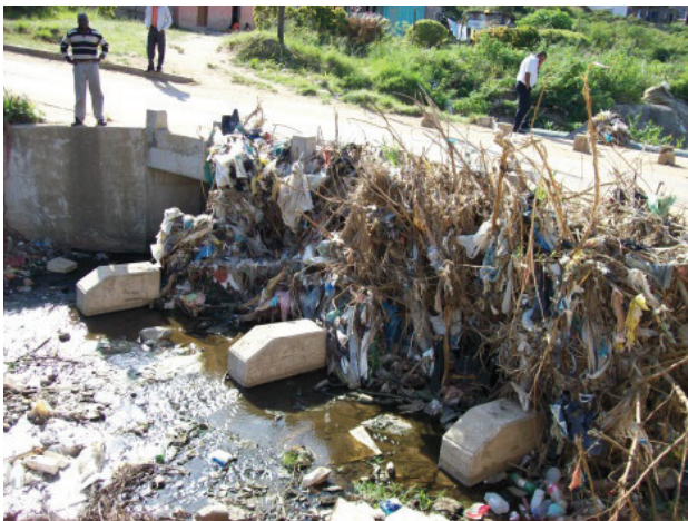
FIGURE 14 Molife Road debris walls and blockage of the culvert
