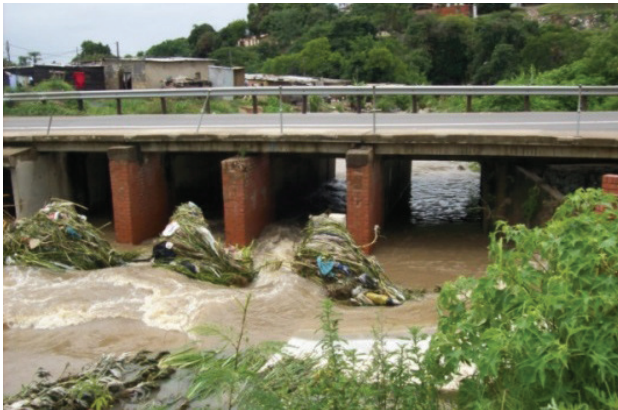
FIGURE 32 Debris walls holding debris - note the acceleration of water towards the centre of the downstream cell
