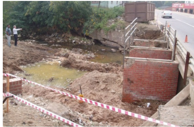
FIGURE 19 The upstream silt in the process of being removed
