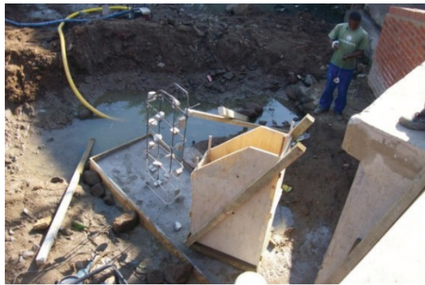
FIGURE 26 Formwork for the debris walls
