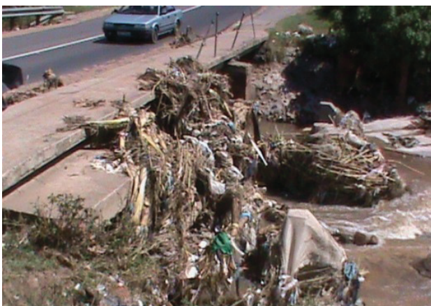
FIGURE 36 Debris build up while the one debris wall was missing
