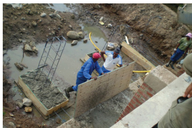
FIGURE 24 Casting of the bases for the debris walls
