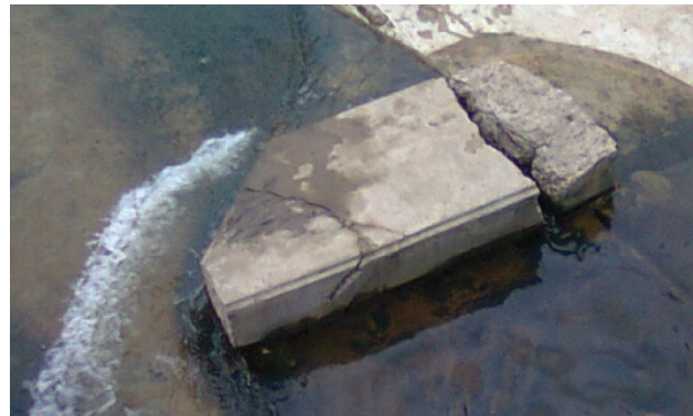
FIGURE 35 Debris wall broken by excavator during the clearing of the debris
