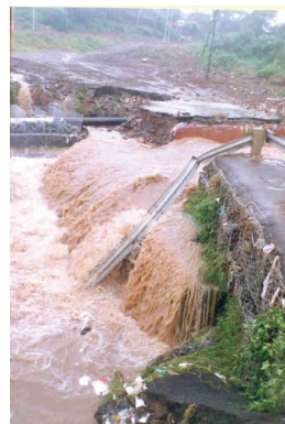
FIGURE 5 The debris deposited upstream of a blocked culvert crossing
