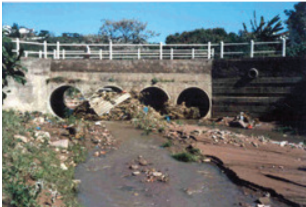
FIGURE 1 Typical blockage of a multicellular pipe culvert after a storm event
