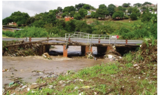
FIGURE 15 Mugabe Road culvert with debris build up
