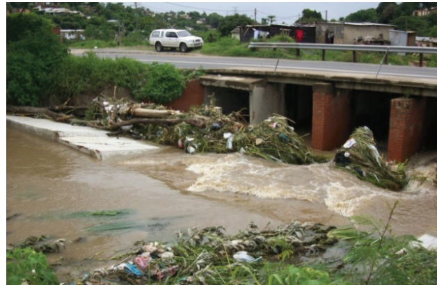
FIGURE 33 Debris including a large tree trunk collected by the debris walls - note that there is no debris on the culvert centre walls
