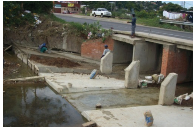
FIGURE 29 Completed debris walls
