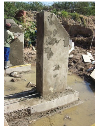
FIGURE 27 Debris walls cast
